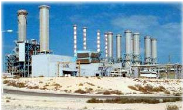
Jebel Ali Desalination Station, Dubai
